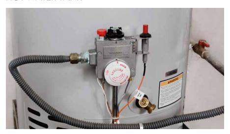
A storage gas-fired water heater is the most common type of appliance used to heat water in Alberta homes. These water heaters typically have a burner at the base and a glass or metal-lined tank. Controls at the base allow you to adjust the temperature and shut down or start up your tank. Most tanks have pilot lights (a small flame that burns continuously) that light the burner when the tank calls for heat. Some tanks have an electronic ignition.
