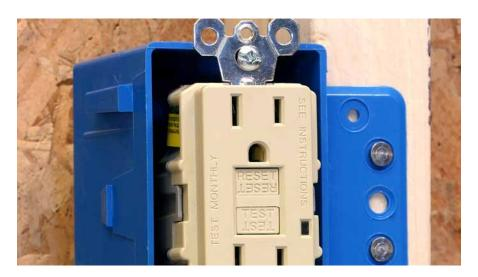
A Ground Fault Circuit Interrupter (GFI) protects people from electric shock. You can recognize a GFI outlet by the 'Test' and 'Reset' buttons located between the plug receptacles of the outlet. One GFI can be wired to protect several electrical outlets on the same circuit.
