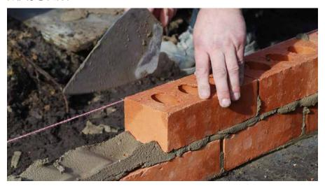
Masonry refers to the stacking of bricks or stones bound together by mortar to create a wall. Clay bricks, concrete bricks, natural stone or many types of manufactured stone available on the market are used in masonry. Masonry veneer walls, a non-structural brick/stone wall laid in front of a structural wall, are made of brick or stone laid in a mortar bed and anchored by metal ties to the wood frame of the home.
