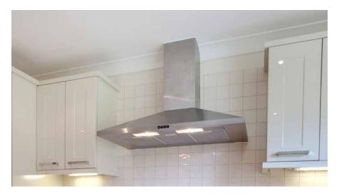
Kitchen range hoods are an important part of your home's ventilation system. They remove odours and improve indoor air quality. Cooking also generates significant airborne moisture which can cause window condensation and mould. A range hood helps draw this moisture out of the home.
